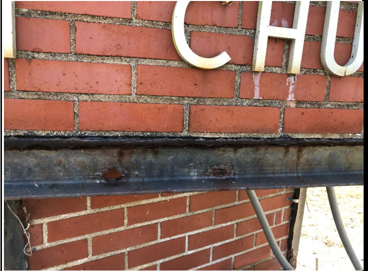
Photo 6: Additional example of corrosion at bell tower monument.
