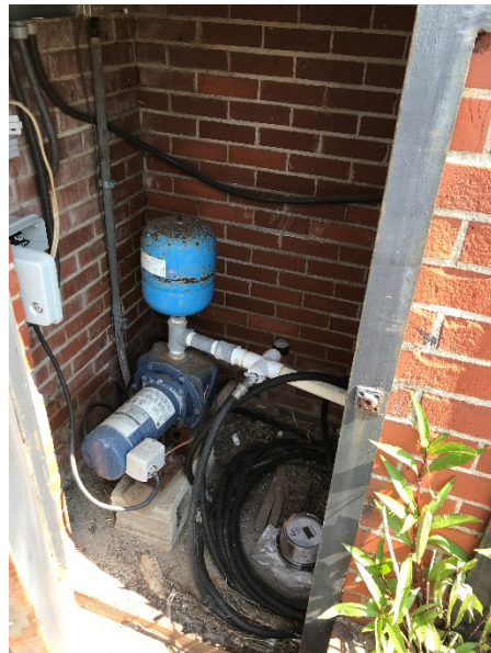
Photo 8: Destroyed irrigation system pump and motor.
