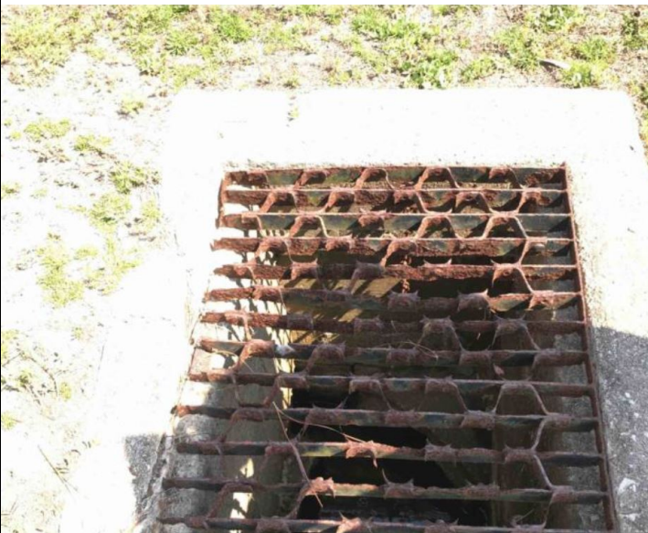
Photo 11: Metal grate drainage structure – connects to off-property drainage collection system.
