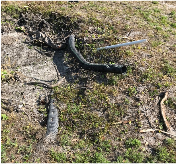
Photo 9: Portion of damaged drainage and irrigation systems.
