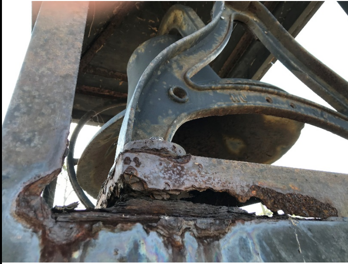
Photo 5: Corrosion severely exacerbated by Hurricane Michael.
