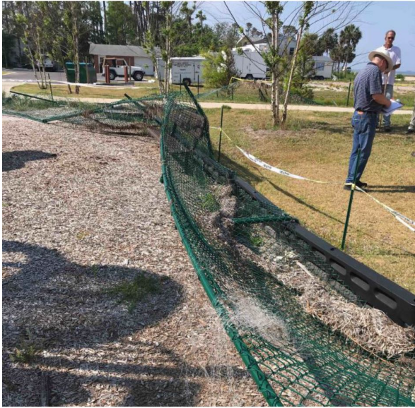
Photo 5: Damaged fence (mid-section of Bayside Playground).
