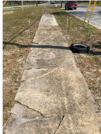
Photo 2: Damaged concrete sidewalk.
