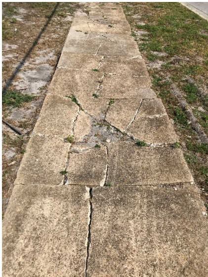
Photo 3: Damaged concrete sidewalk.
