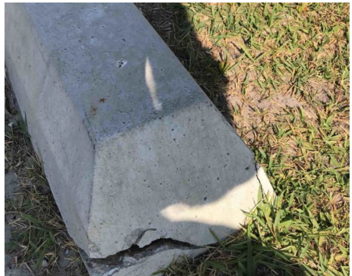
Photo 4: Damaged concrete curb (car parking stop).
